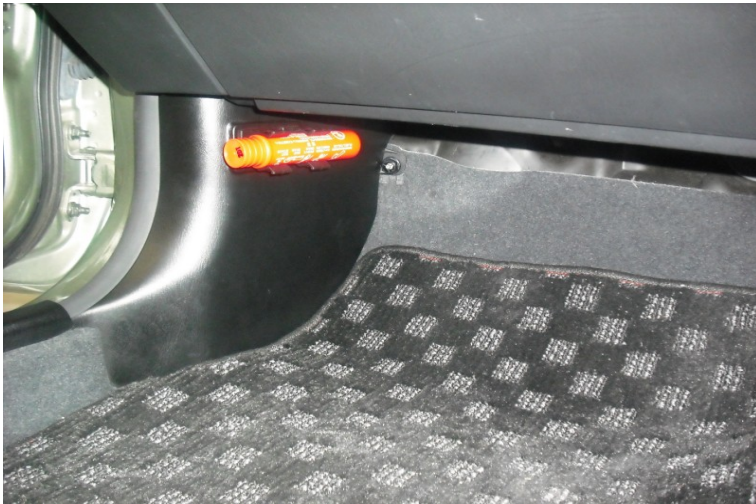
Figure 1 – Left hand side kick panel showing ECU Location
